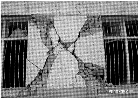
图 1 墙体的贯穿 X 形裂缝 Fig. 1 X-shape cracks on the wall
