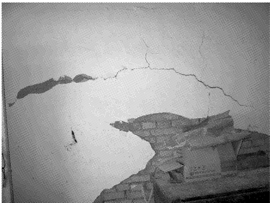
照片8 西吉县兴平乡一户房屋墙体开裂 Photo 8 Wall cracks in Xingping Village, Xiji County
