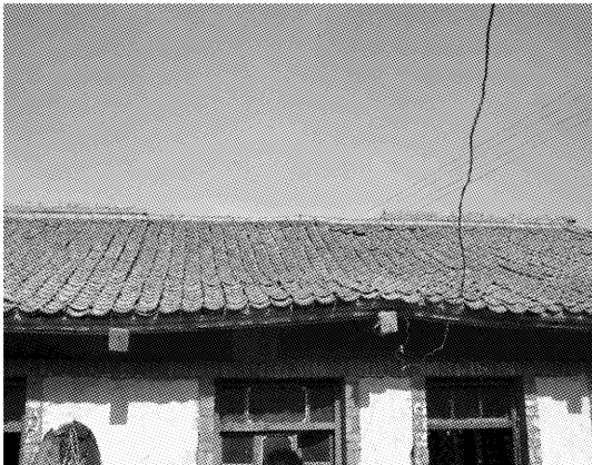
照片7 泾源县泾河源镇一户房屋 屋脊掉落和屋顶变形 Photo 7 Fastigium flopped and roof shaped in Jinghe Town, Jingyuan County
