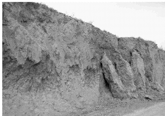
照片 1 隆德县观庄乡乡间土路旁黄土崩塌 Photo 1 A loess collapse of rural road-side in Guanzhuang Village, Longde County
