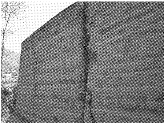
照片9 海原县郑旗乡一户房屋墙体外闪 Photo 9 An outward-leaning wall in Zhengqi Town, Haiyuan County
