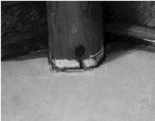
照片6 彭阳县城阳乡一户房屋横梁错位 Photo 6 Beam movement in Chengyang Village, Pengyang County
