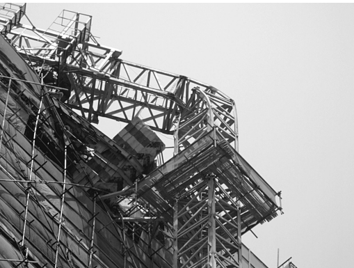
图 3 西安市一建设工地正在施工的塔吊折断 Fig 3 A tower crane broke in operation at a construction site in Xi'an
