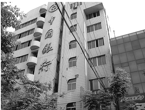
图 5 宝鸡市陈仓区东西大街中国银行大楼破坏 Fig 5 Damage of a building of Bank of China in the Dongxi street in Chencang District of Baoji City
