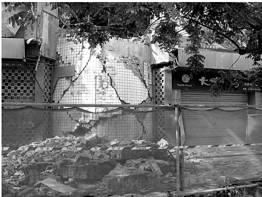
图 4 宝鸡市陈仓区东西大街某转角楼破坏严重 Fig 4 Heavy damage of a corner house in the Dongxi street in Chencang District of Baoji City
