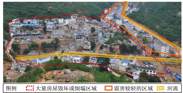
图 1 宏观震中龙头山镇建筑震害情况 Fig. 1 Seismic damage of the macro epicenter, Longtoushan town
