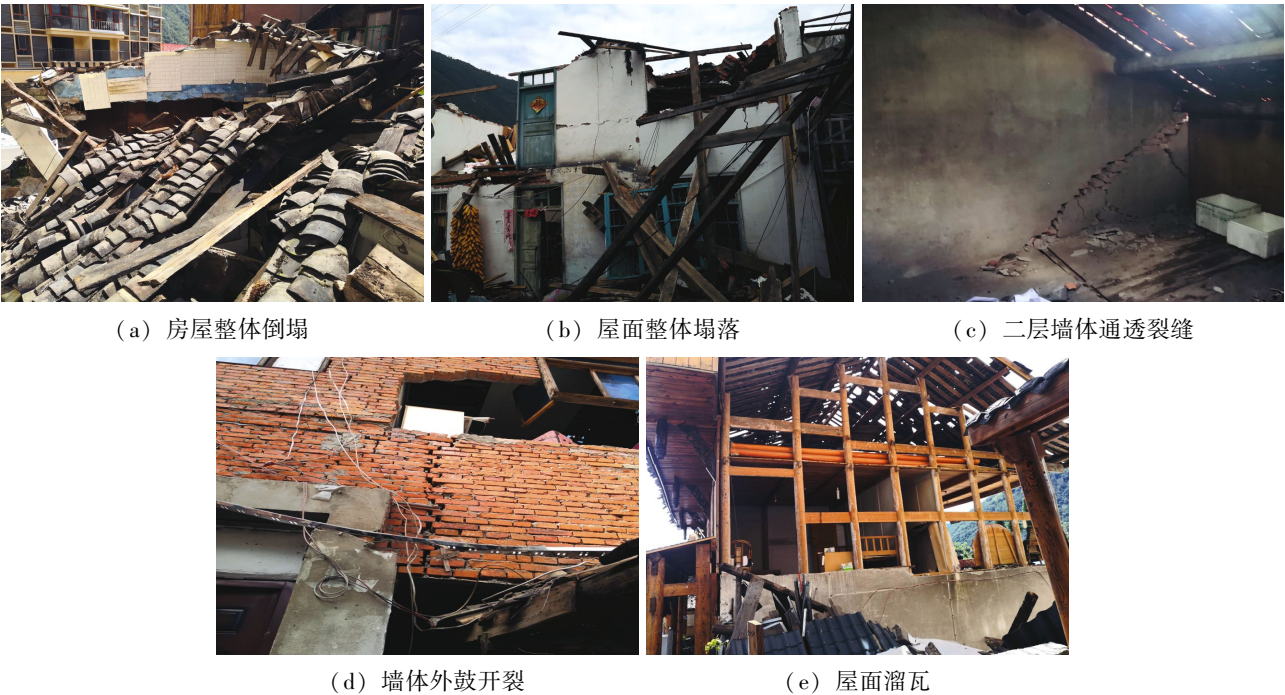
图 4 砖（石）木房屋典型震害 Fig. 4 Typical seismic failure of masonry and wood structure buildings
