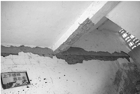
图 6 德化中学砖混教学楼破坏 Fig 6 Brick & Concrete building destroyed in Dehua Middle School
