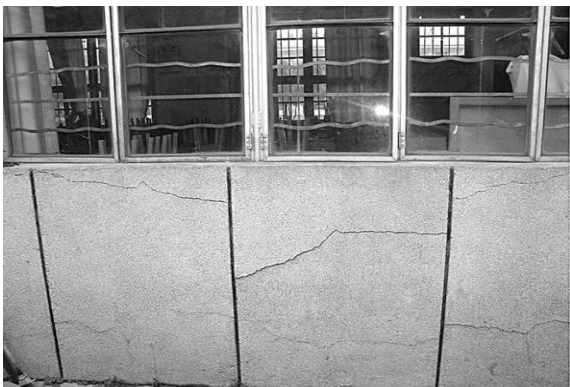
图 7 正兴中学框架教学楼窗肚墙开裂 Fig 7 Cracks on the wall of frame building in Zhengxing Middle school
