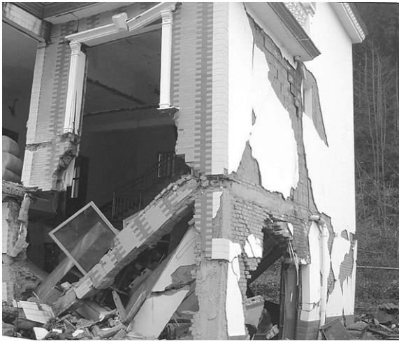
图 8 构造柱与圈梁受力失效 Fig 8 Loading failure of constructional column and ring beam
