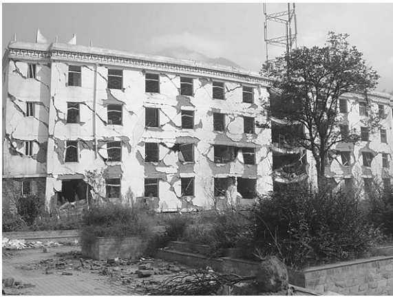
图 11 映秀镇漩口中学宿舍楼剪切破坏 Fig 11 Dormitory of Yingxiu Middle School suffered shear damage
