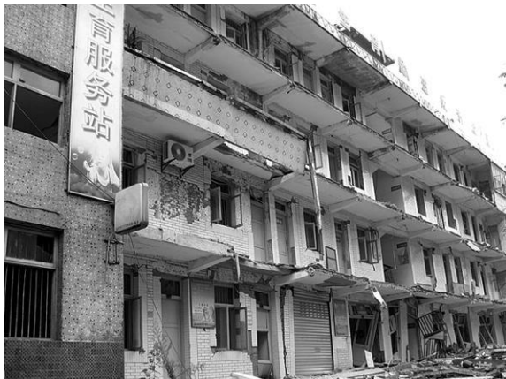
图 12 北川县计生服务站办公楼外走廊栏杆倒塌 Fig 12 Brick fence in outside corridor of office building collapsed
