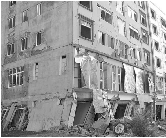
图 10 底层框架砖混结构发生严重破坏 Fig 10 Brick-concrete structure of bottom frame was seriously damaged
