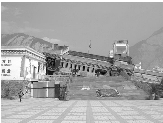
图 9 “强梁弱柱”类型的破坏案例 Fig 9 Damage case of strong beam and weak column
