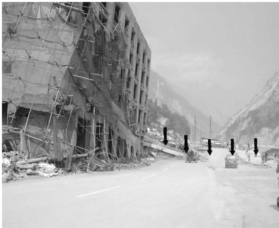
图 2 映秀公路旁在建建筑物结构严重破坏 Fig 2 Buildings under construction beside Yingxiu Road was severely damaged
