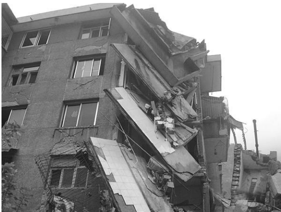
图 7 预制板引发的多米诺骨牌效应 Fig 7 Domino effect triggered by prefabricated slabs
