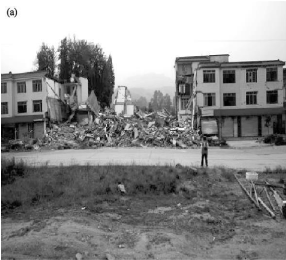
图 2 映秀公路旁在建建筑物结构严重破坏 Fig 2 Buildings under construction beside Yingxiu Road was severely damaged
