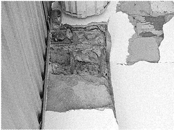
图3 星星佳园框架房屋的柱子上部钢筋弯曲外露 Fig. 3 Pillars of the upper frame house exposed steel bending in Xingxing Residential Quarter
