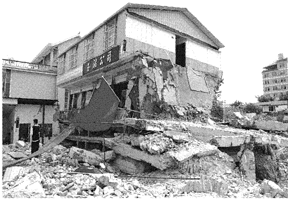
图5 玉锦公司三层砖混楼的一、二层坍塌 Fig. 5 First and the second floor of a brick-concrete and three-story building of Yujin Company collapsed
