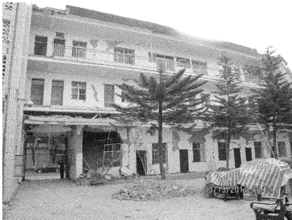
图6 盈江县国土局砖混办公楼毁坏 Fig. 6 Brick-concrete building of Yingjiang County Land Resource Bureau destroyed
