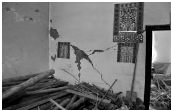
图9 水墨镇嵩坪村土木结构房屋垮塌 Fig. 9 Civil structure building collapse in Songping Village, Shuimo Town
