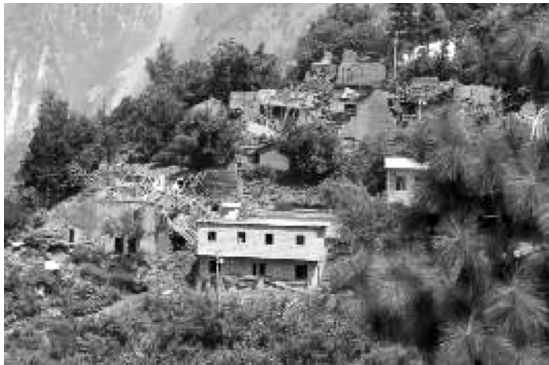
图5 巧家县包谷埡乡老屋基村土木结构房屋倒塌 Fig. 5 Civil structure building collapse in Laowuji Village, Baogunao Township, Qiaojia County
