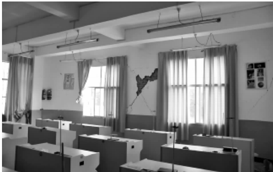
图 12 鲁甸县城砖混结构教学楼“X”型裂缝 Fig. 12 “X” cracking of the wall of brick-concrete structure building in Ludian Town
