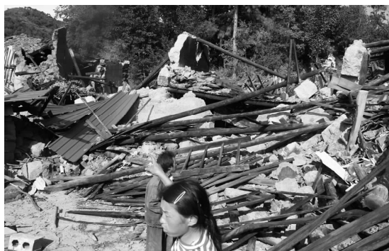
图8 火德红镇银厂村土木结构房屋倒塌 Fig. 8 Civil structure building collapse in Yinchang Village, Huodehong Town
