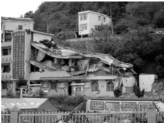
图3 龙头山镇中学砖混结构房屋毁坏 Fig. 3 Brick-concrete structure building destroy in Longtoushan Town middle school
