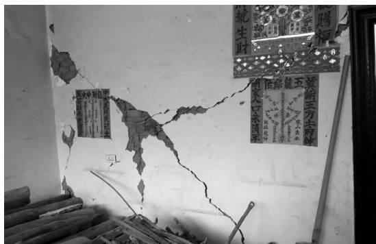
图10 文屏镇安阁村砖混结构房屋“X”型裂缝 Fig. 10 “X” cracking of the wall of brick-concrete structure building in Ange Village, Wenping Town
