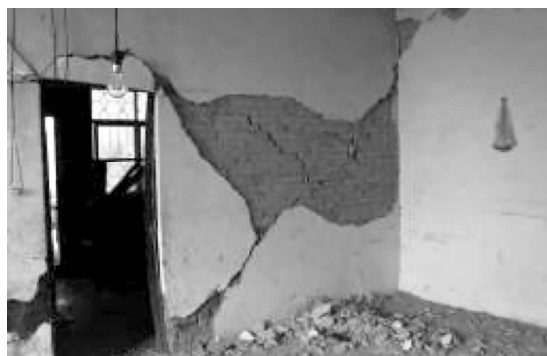
图7 龙头山镇沙坝村砖混结构房屋墙体“X”型裂缝 Fig. 7 “X” cracking of the wall of brick-concrete structure building in Shaba Village, Longtoushan Town
