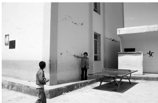
图6 火德红镇李家山村框架结构房屋墙体开裂 Fig. 6 Wall cracking of frame structure building in Lijiashan Village, Huodehong Town
