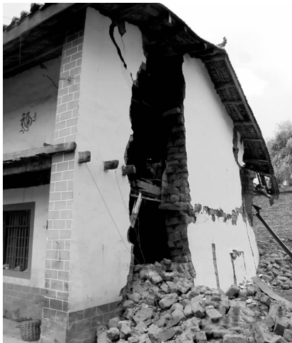
图 13 昭阳区苏甲乡土木结构局部垮塌 Fig. 13 Civil structure building locally collapse in Sujia Village, Zhaoyang Area
