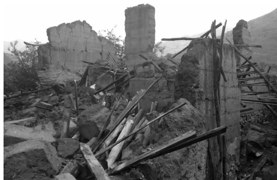
图11 会泽县纸厂乡土木结构房屋垮塌 Fig. 11 Civil structure building collapse in Zhichang Village, Huize Town
