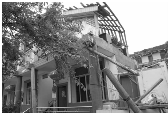
图 4 芦山河岸边砖混结构房屋严重破坏 Fig. 4 Serious destruction of brick concrete building in the side of Lushan River
