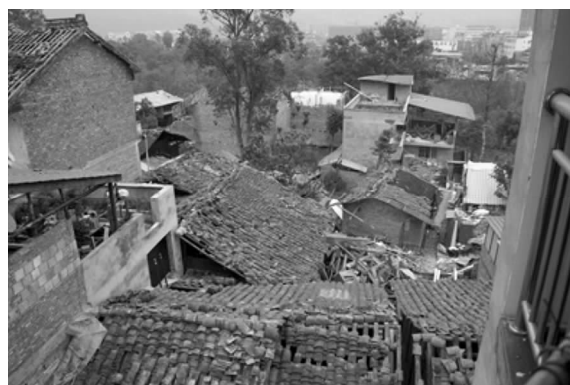
图10 房顶瓦片掀翻 Fig. 10 Tiles of roof tilting
