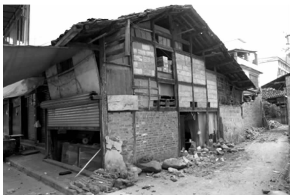
图9 砖木结构房屋严重破坏 Fig. 9 Serious destruction of brick wood building
