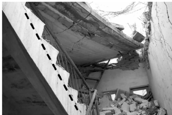
图 6 楼梯间现浇混凝土楼板倒塌 Fig. 6 Collapse of cast-in-place concrete floor in the stairs
