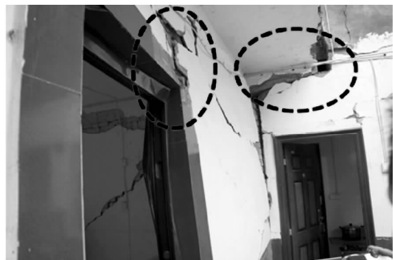
图 5 砖混结构房屋墙体位移 Fig. 5 The deformation of wall of brick concrete building
