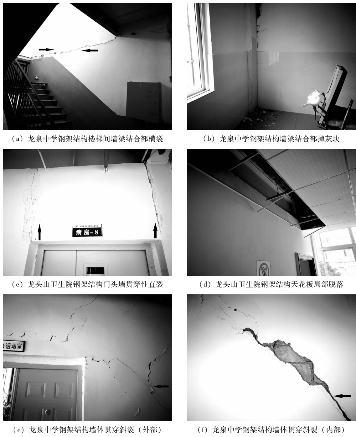
图 7 钢架结构房屋震害特征 Fig. 7 Earthquake damage characteristics of steel frame structure building
