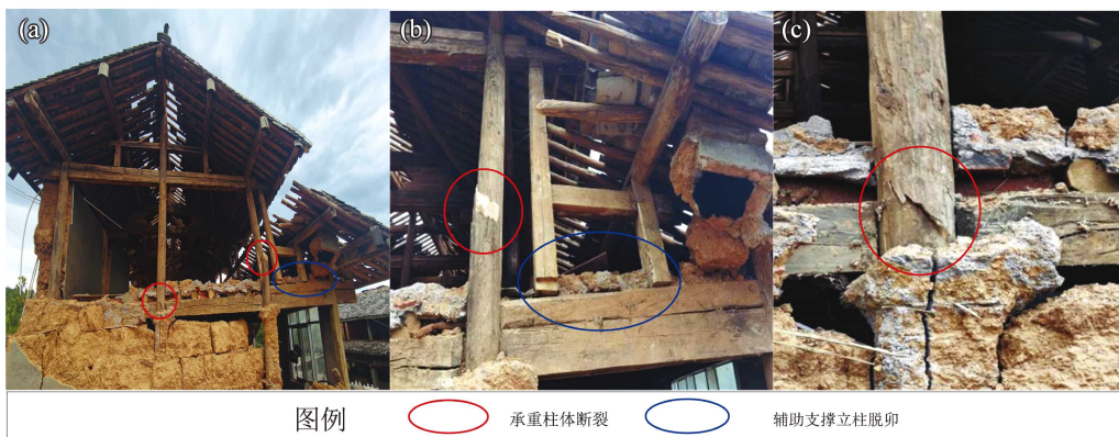
图5 居住房左侧第一间柱和梁破坏情况 Fig. 5 Damage to the pillars and beams of the 1st room on the left of the Main house
