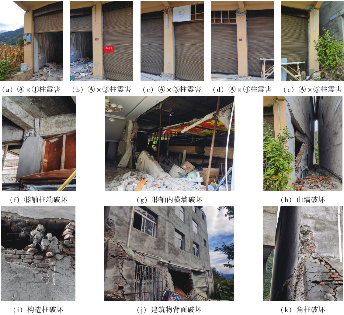
图 10 大杉树村 6 组 56 号建筑一层震害图 Fig. 10 Seismic damage to the first floor of No. 56 building in Group 6 of Dashanshu Village
