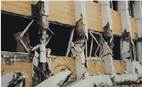
(e) 汶川地震中框架结构框架柱脆性剪切破坏
