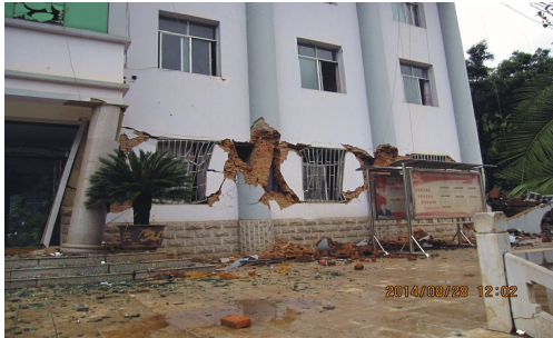
(c) 鲁甸地震中砌体结构砖柱剪切破坏
